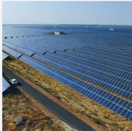
300MWp+126MWh Solar-Storage turnkey EPC, CIS region
