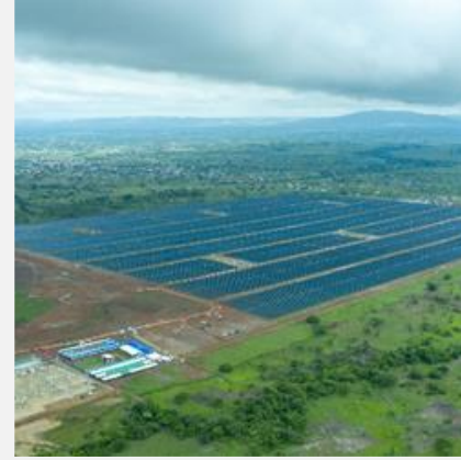
50MWp Solar PV turnkey EPC, West Africa
